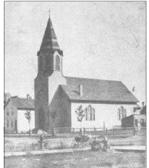
St. Peder's first church at 20 th Avenue South and 9 th Street South.
